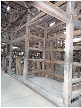
FIGURE 9. Kominka house (Nago, 1906)
