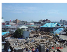
(a) Total Collapse
