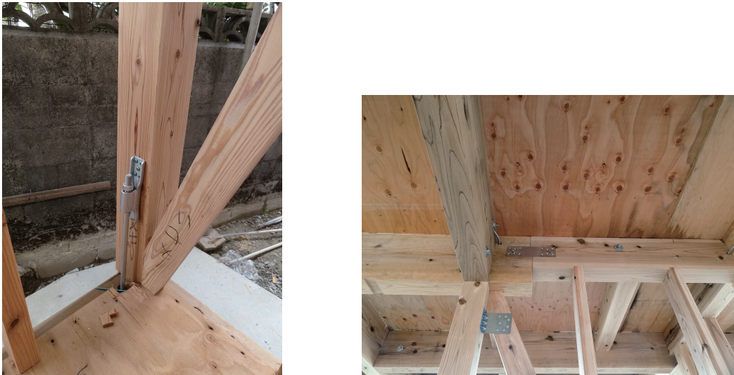
FIGURE 15. Steel connectors in wooden houses
