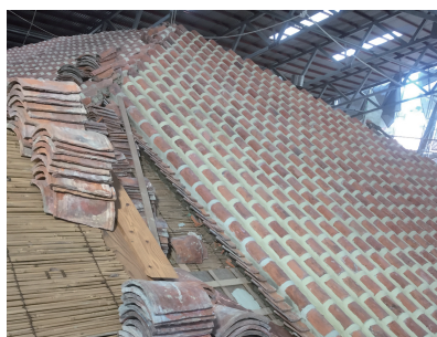
FIGURE 8. Red tile roof under repair
